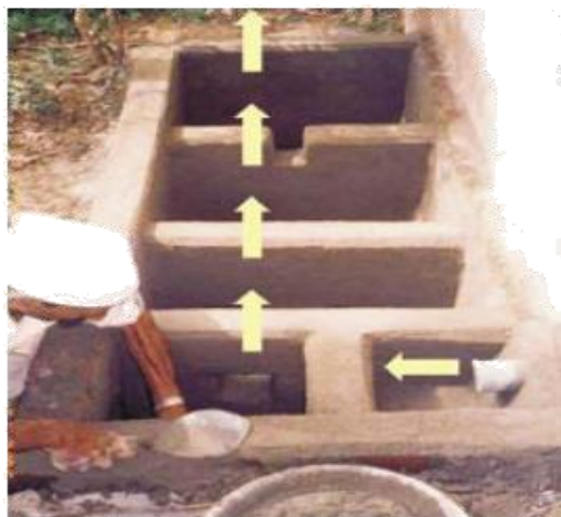
Construction of greywater treatment system
