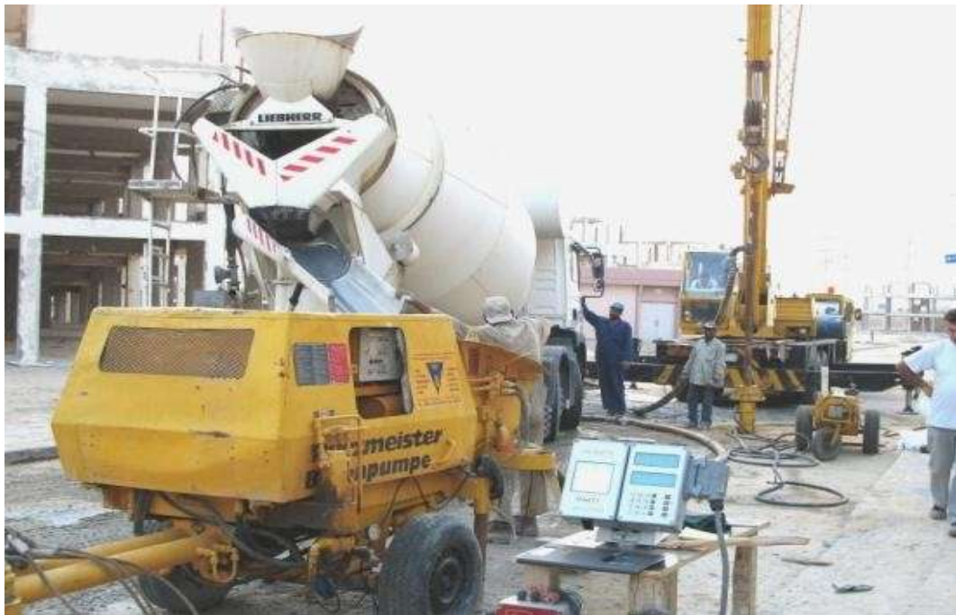
Figure2: Deliveryofcavityfillingmix
