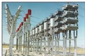
Figure-2: Shunt capacitor bank at grid substation
