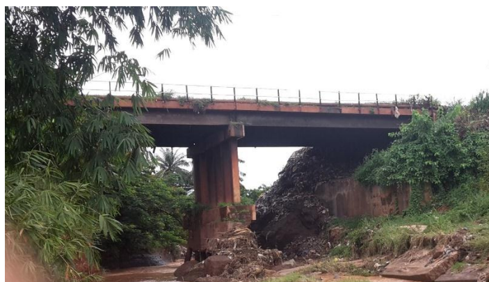
Figure 3.1: The Abakpa Bridge along Nike Road, Enugu
