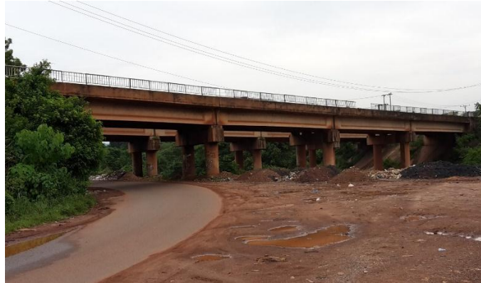
Figure 3.2: The Abakpa fly-over bridge, at 82- Division axis along the Enugu-Onitsha Express
