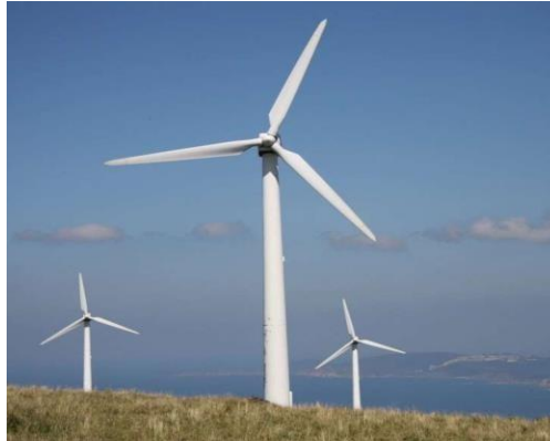
Fig.3. NEG Micon 1.5MW Wind Turbine, 68m diameter Rotor, Tubular Steel Tower. Blades are made up of fibreglass. The Rotor blades can be Turned to optimise power & the entire tower is rotated to face the wind.
