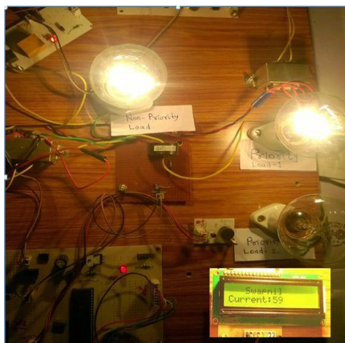
Fig.8. Full load condition of Transformer
