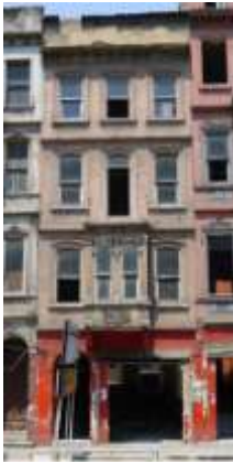
Figure 5. The construction facade viewing the Tarlabası Boulevard
