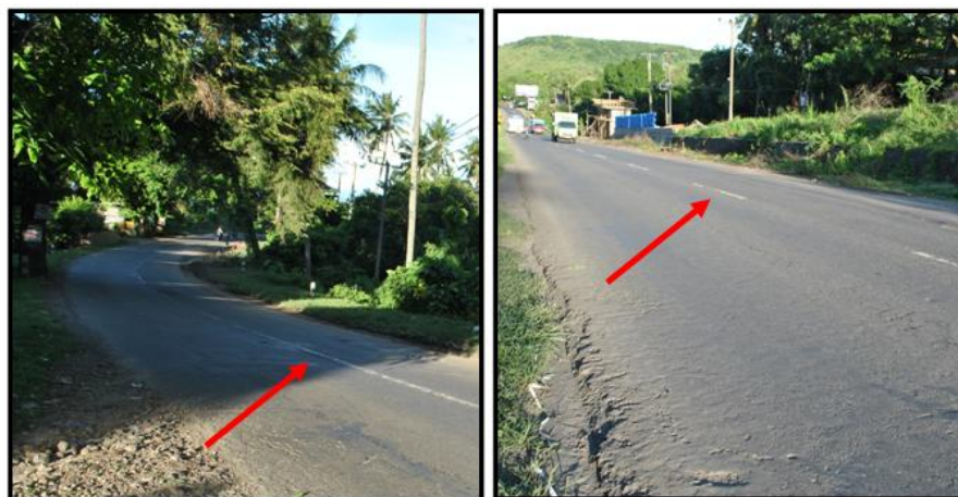
Figure 4. Longitudinal Mark intact lines and dotted
