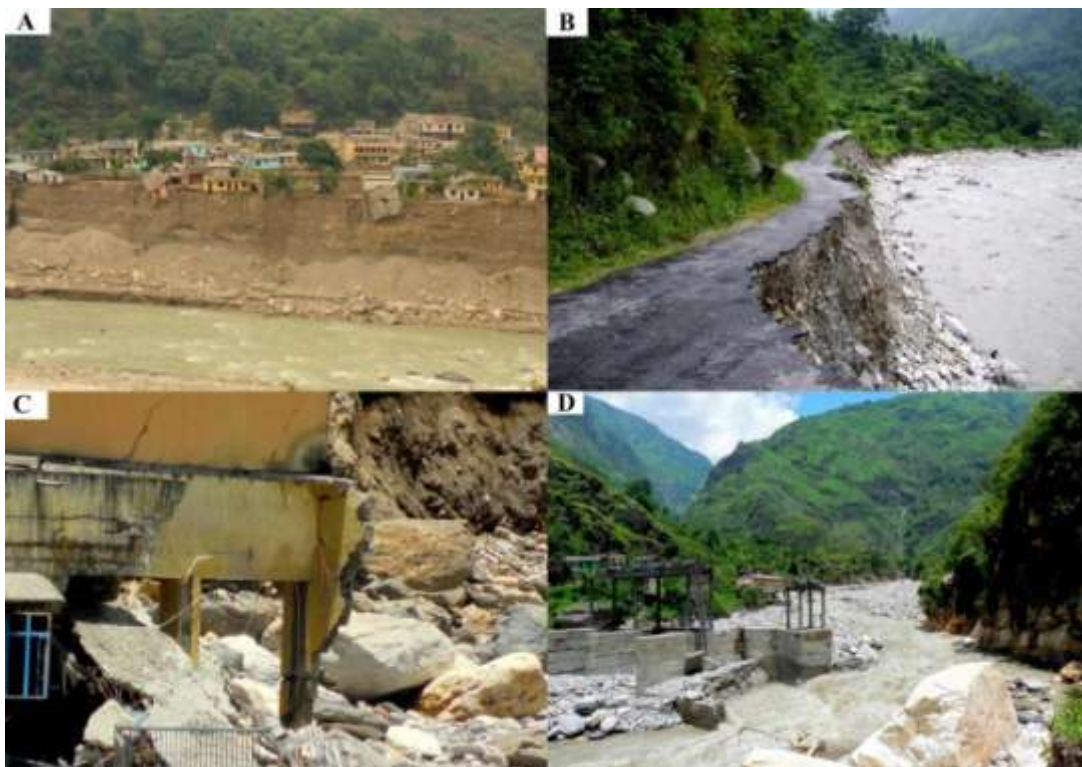
Plate-2: Impact of flash flood and mass wasting disasters in district Pithoragarh: (A) at Ghatta Bagar (2013), (B) at Morivillage (2013), (C) at Dani Bagar (2016) and (D) Himalaya Hydro Power Project Dam damaged at Bali Bagar (2018) (based on field survey).
