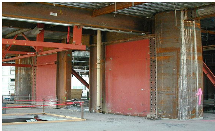
Figure 11: Coupled steel plate shear wall [9].
