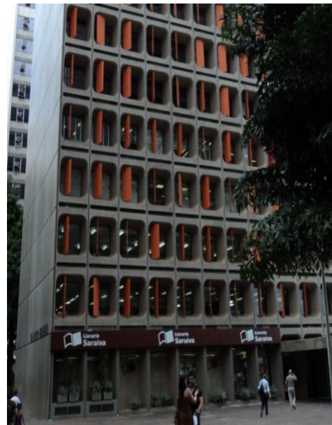
Figure 3 - mobile Brises (ARAÚJO, SIMÕES & SPOSTO, 2012)
