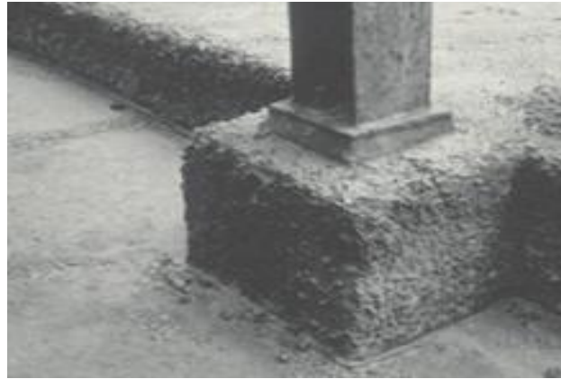
Fig 2 Severity of sulphate attack depends on type and concentration of the sulphate and increases with wetting and drying
